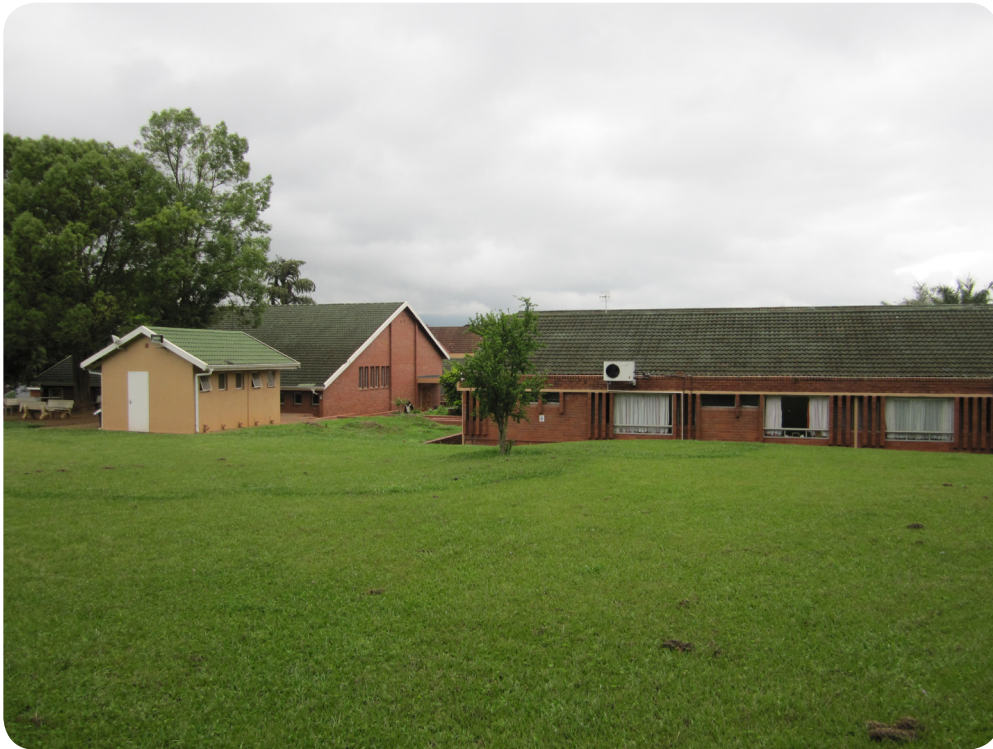
The existing residential facility on the site
